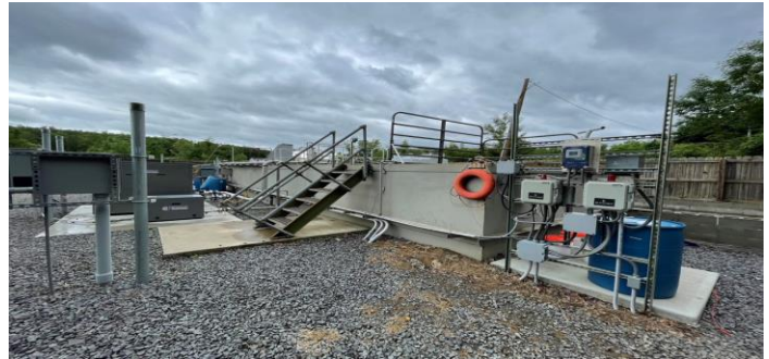
After – Overhaul of plant
