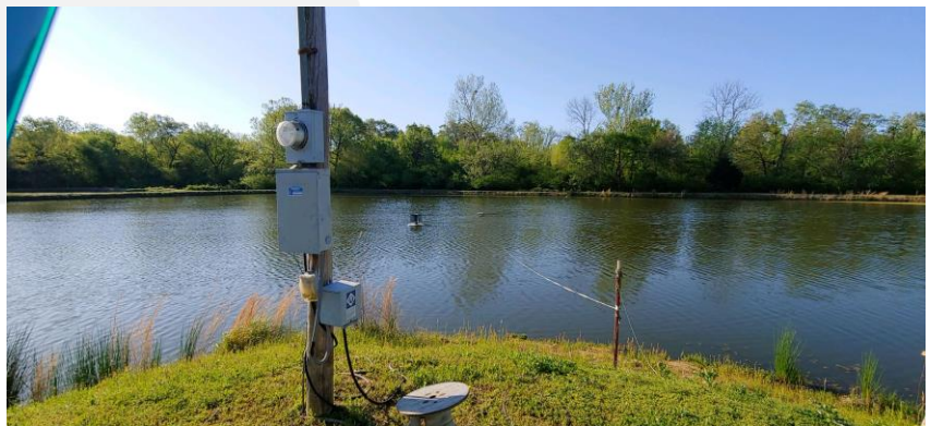
After – Wastewater system improvements
