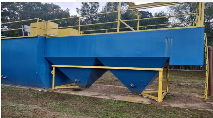
After – Upgrades to facility
