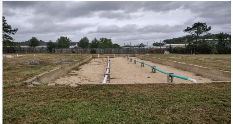
After – Re-piping and clean up of sand filter
